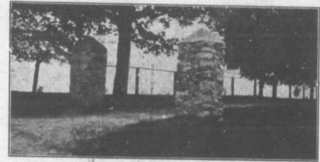
A Farm Entrance One Would Not Soon Forget. These massive columns are simply constructed of ordinary boulders capped with cement. Entrance to the garden home of Albert Jull, Brant Co., Ont.
