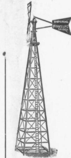
OUR TOWERS are girted every five feet apart, and double-braced. This doubly insures against accidents in storms. All Mills are galvanized after completion. This gives increased strength.
