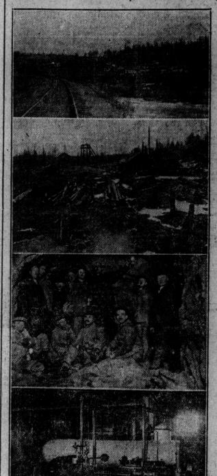
The above are splendid illustrations of the mine as it appears to-day. Note the railway running through, the camp buildings, shaft head, etc. Trains stop right at the mine. Shaft is down 215 feet, cross-cut at 100 ft. level. All the buildings are of substantial
