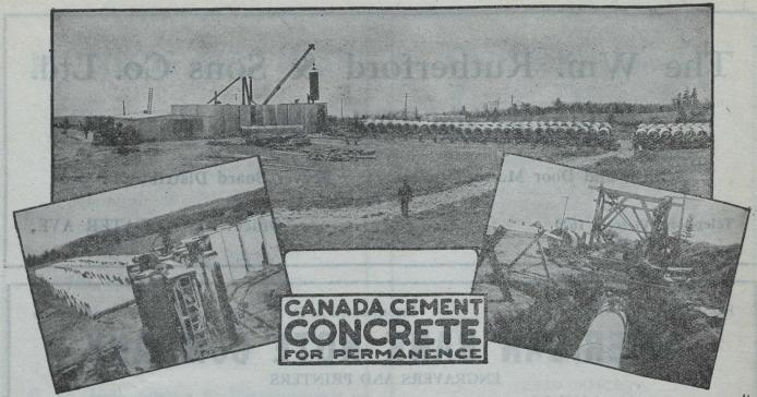
The forms are of steel, held by cast iron top and bottom rings, which insure great accuracy and smoothness of finish.
