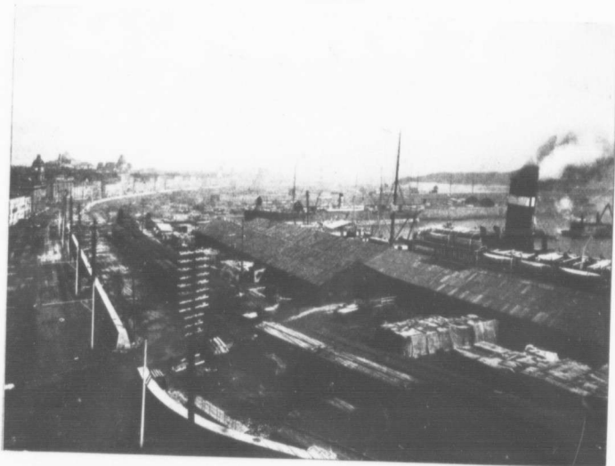
A PORTION OF MONTREAL HARBOR.
