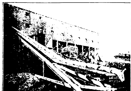
Freight and Package Elevator
