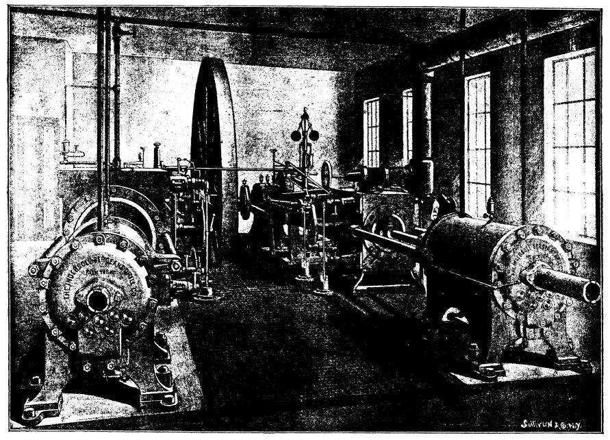
Corliss Cross-Compound. Air Cylinders 22 in. Diameter by 42 in. Stroke.
