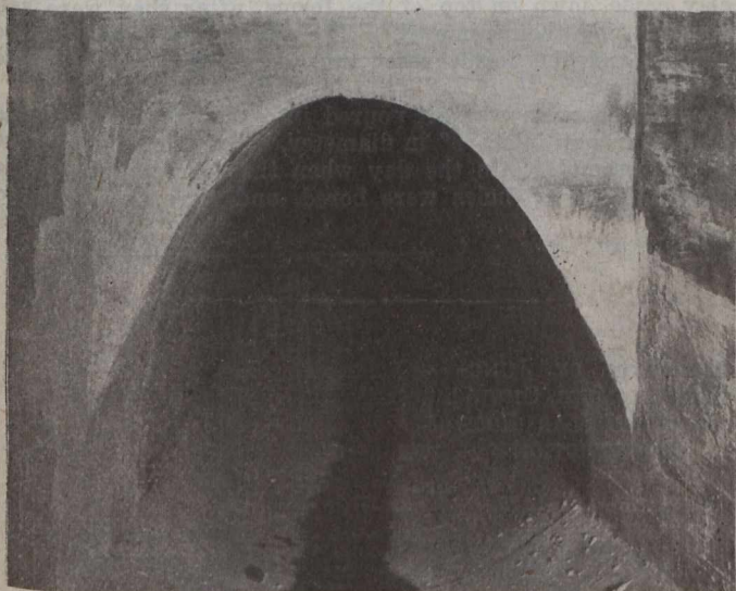
SOUTH END OF JUNCTION CHAMBER, LOOKING INTO COMPLETED SEWER
