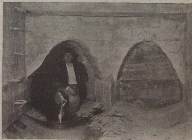
NORTH END OF CHAMBER, WITH CONNECTIONS FOR EAST AND WEST EXTENSIONS
