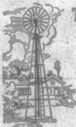
For over thirty years our Windmills have been noted for their wonderful work in light winds. Troughs or water systems don't run dry when supplied by TORONTO Windmills. With this light-wind ability we have combined sturdy strength and self-regulating features that enable Toronto Windmills to stand up to the fiercest gales, and to stop and start themselves when water is needed. Write for our Illustrated Booklet telling all about them. 15
