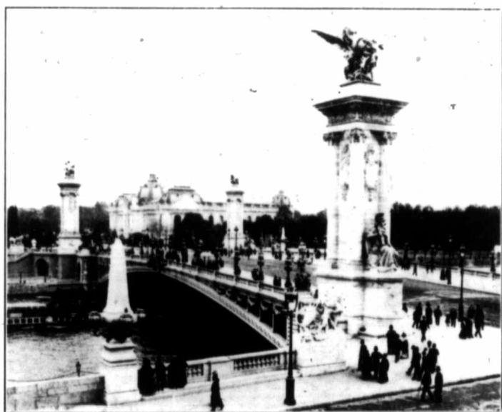
Fig. 3—Alexander III. Bridge, Paris.
