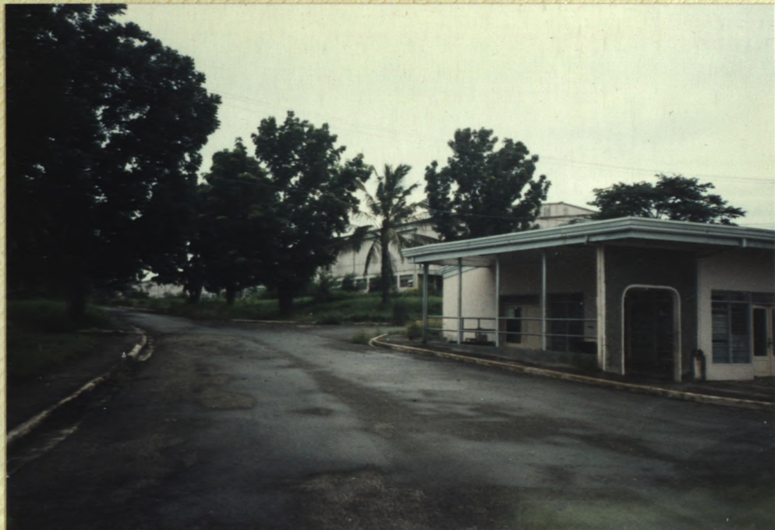
No. 1. Entrance to NHC Complex. Guardhouse and employee time clock station in right foreground. Woodworking plant in background.
