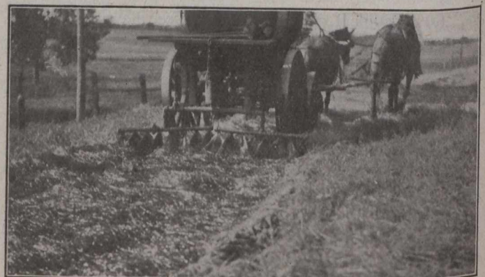
Applying Tar to Straw; First Application
