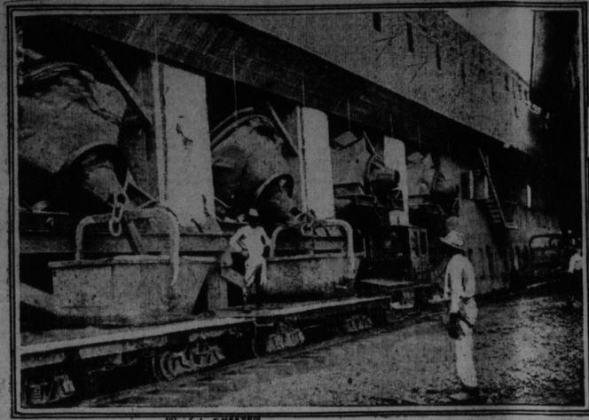
This photograph was taken in the great concrete mixing works on the hilltops overlooking the Gatun dam—it shows one of the batteries of mixers.
