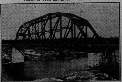
BRIDGE OVER THE PICKEREL RIVER, ON THE C.N.R. LINE TO SUDBURY—SPAN 296 FT.; CENTRE HEIGHT 52 FT.
