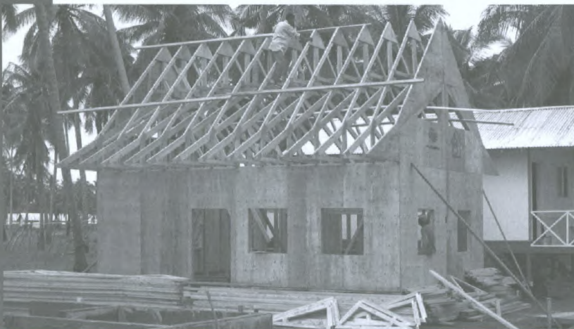
Canadian companies have contributed 10 wood-frame homes to the Labui Eco-Village in Banda Aceh, Indonesia.
