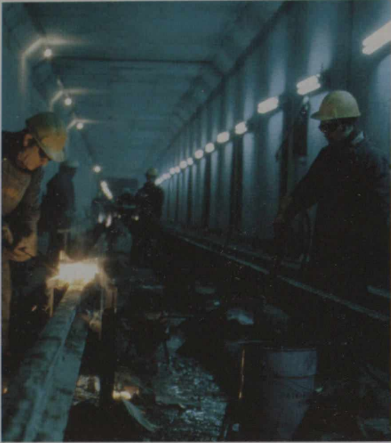
Building the Finch extension of the Toronto subway.
