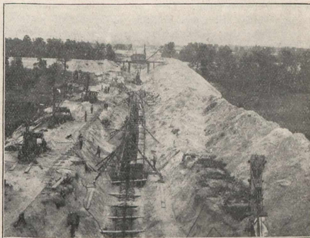
Bird's Eye View of Gary Sewer, Showing Pumping Plant, Trench, Clamshell, Backfilling and New Steel Plant in Far Distance.
