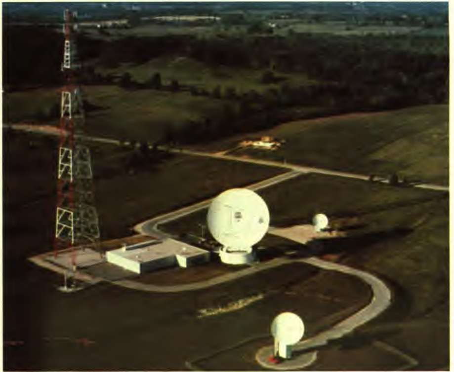
Telesat's two control stations at Allan Park, Ontario, (right and top left) and Lake Cowichan, British Columbia, (bottom left) have 30-metre antennas. The three smaller antennas at Allan Park provide tracking, telemetry and command functions. The satellite control system developed by Telesat has been used in the United States, Indonesia and Brazil.
