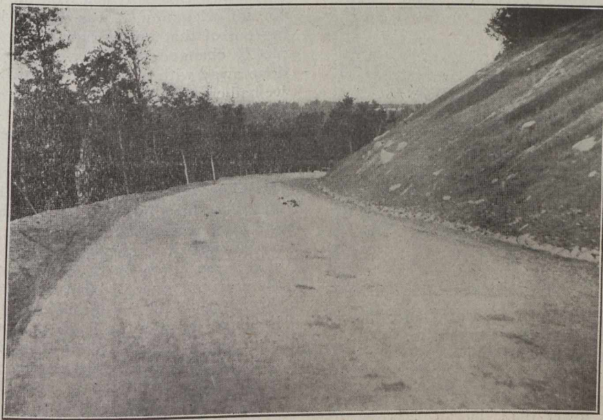
Fig. 1.—Montreal-Quebec Road, Donnacona (Portneuf). Macadam Done in 1915.
