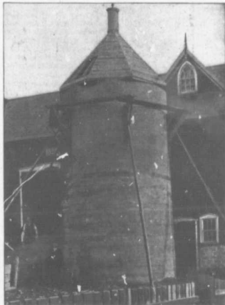
A CEMENT SILO 16 FT. X 35 FT.
