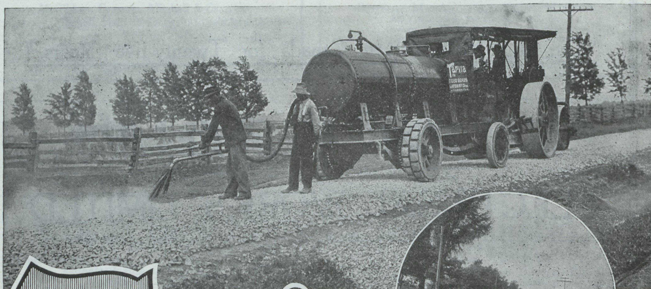
Applying "Tar via" X" on Ken- nedy Road, Scarboro Township, Ont. Toronto and York Roads Commission. The view in the circle is the finished road. Note smooth, dustless surface.
