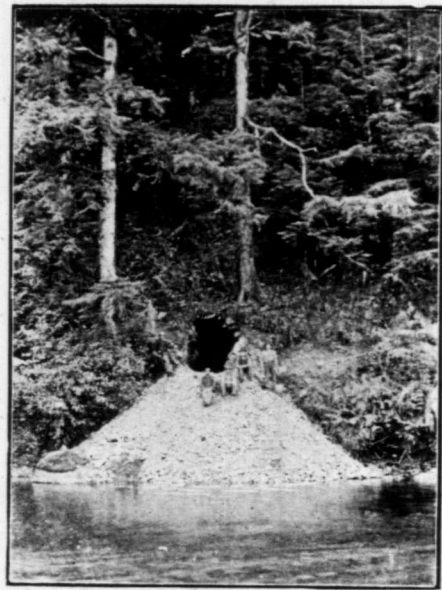
MOUTH OF TUNNEL, SARITAS RIVER.
