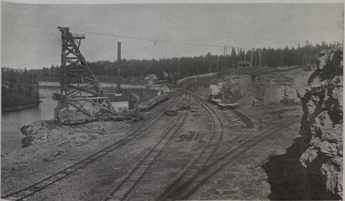
General View of Quarry Yard, Showing Track Layout, Cableway and Rock Formation.
