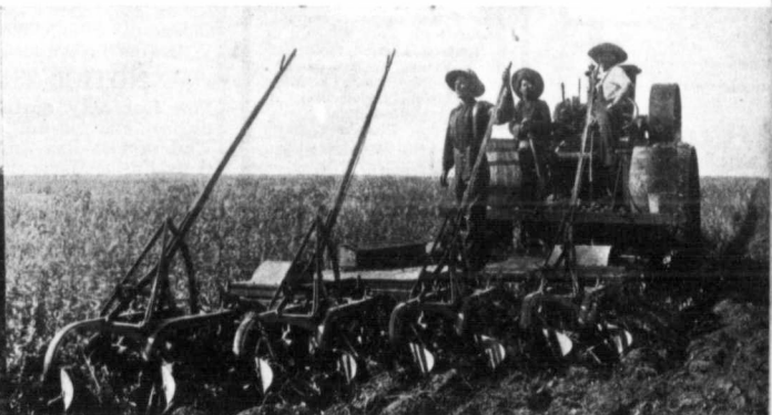
A Sawyer and Massey Combination Plowing Engine pulling the 8 bottom 14 inch John Deere Engine gang Outfit of Jones Bros., Whitewater, Man.
