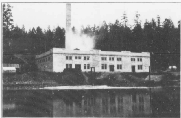
Brentwood Steam Plant
