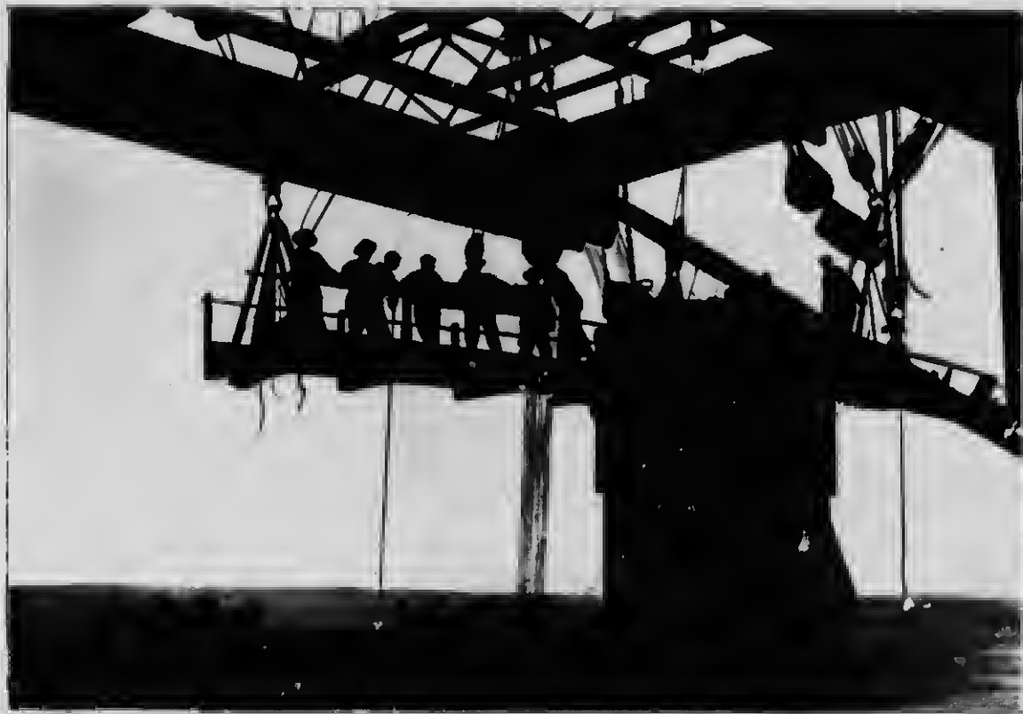
DRIVING A 12-INCH TOP CHORD PIN.
