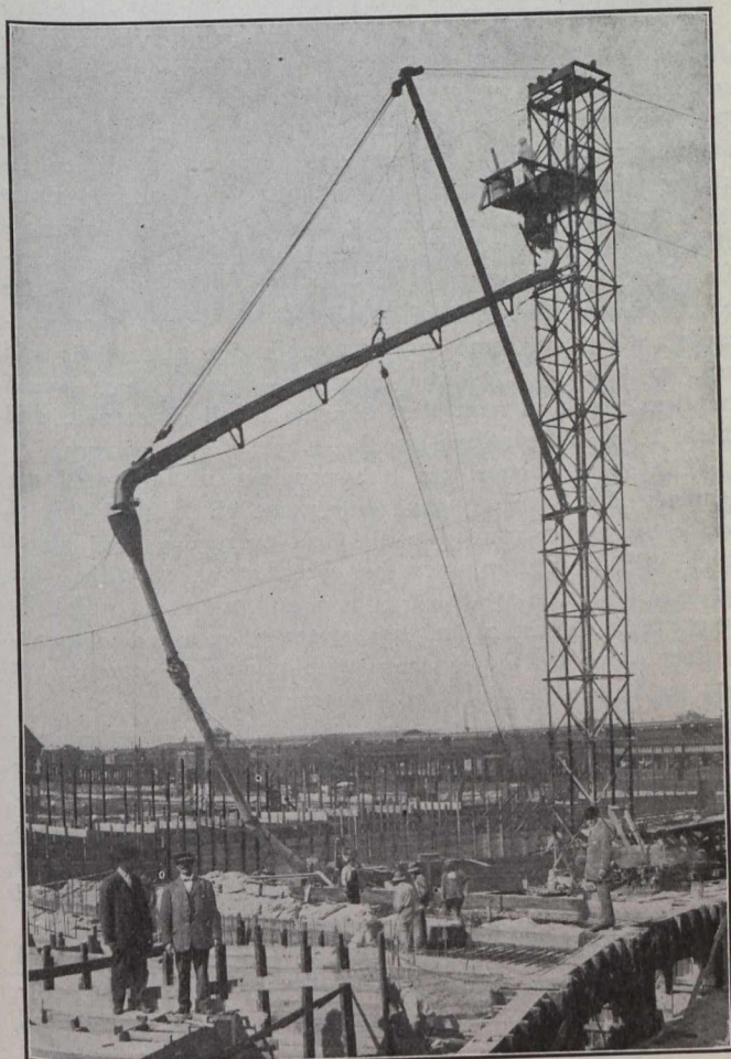
Fig. 2.—View of Steel Tower, Showing Concrete Chute in Position.
