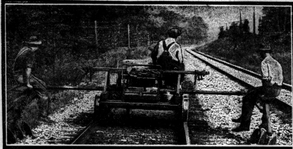
Railroads have installed motor plows that serve the double purpose of cutting the weeds and leveling the ballast on the road. This work was formerly done by hand.
