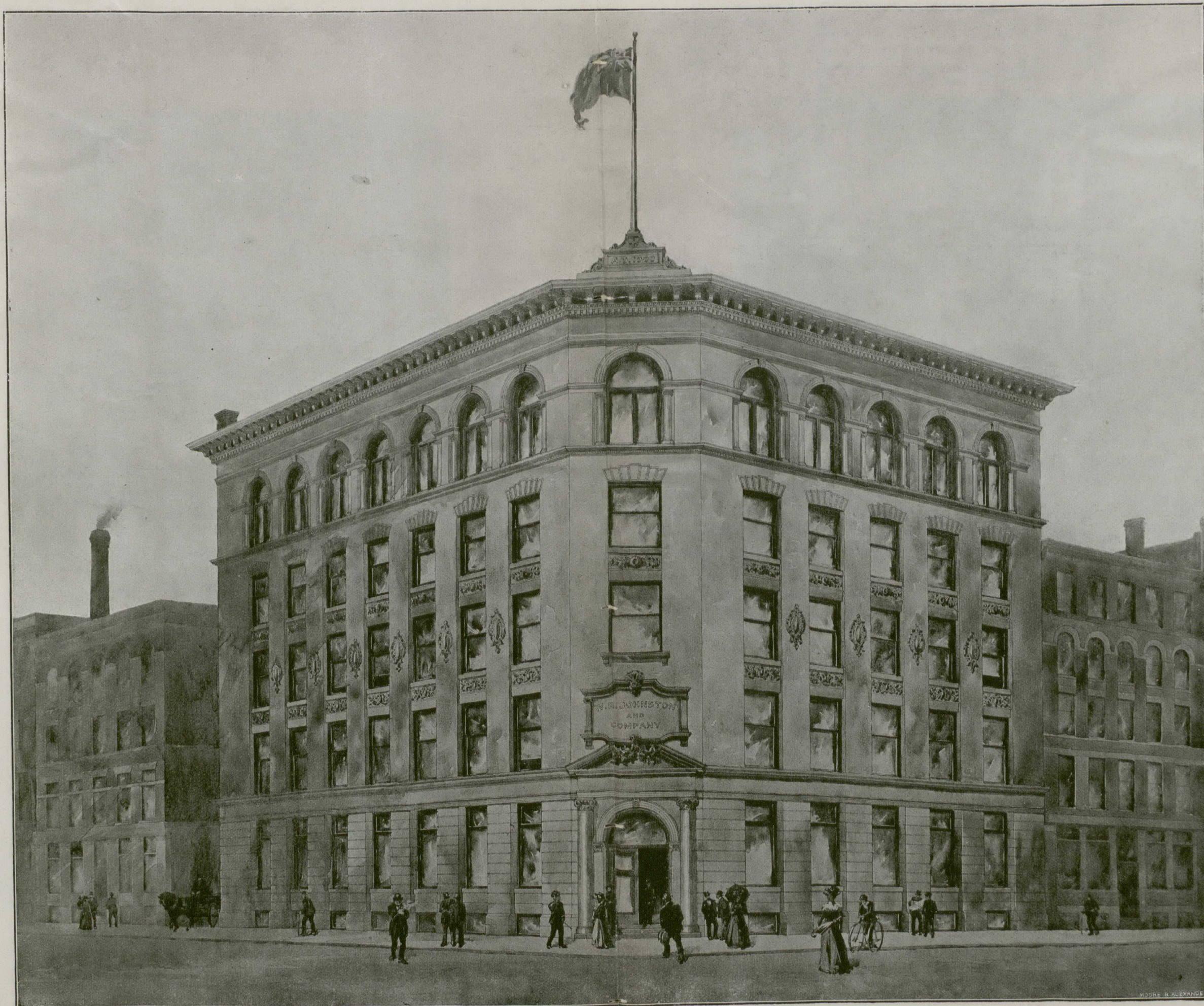
WAREHOUSE FOR MESSRS. W. R. JOHNSTON & COMPANY, FRONT STREET, TORONTO. MESSRS. GORDON & HELLIWELL, ARCHITECTS.
