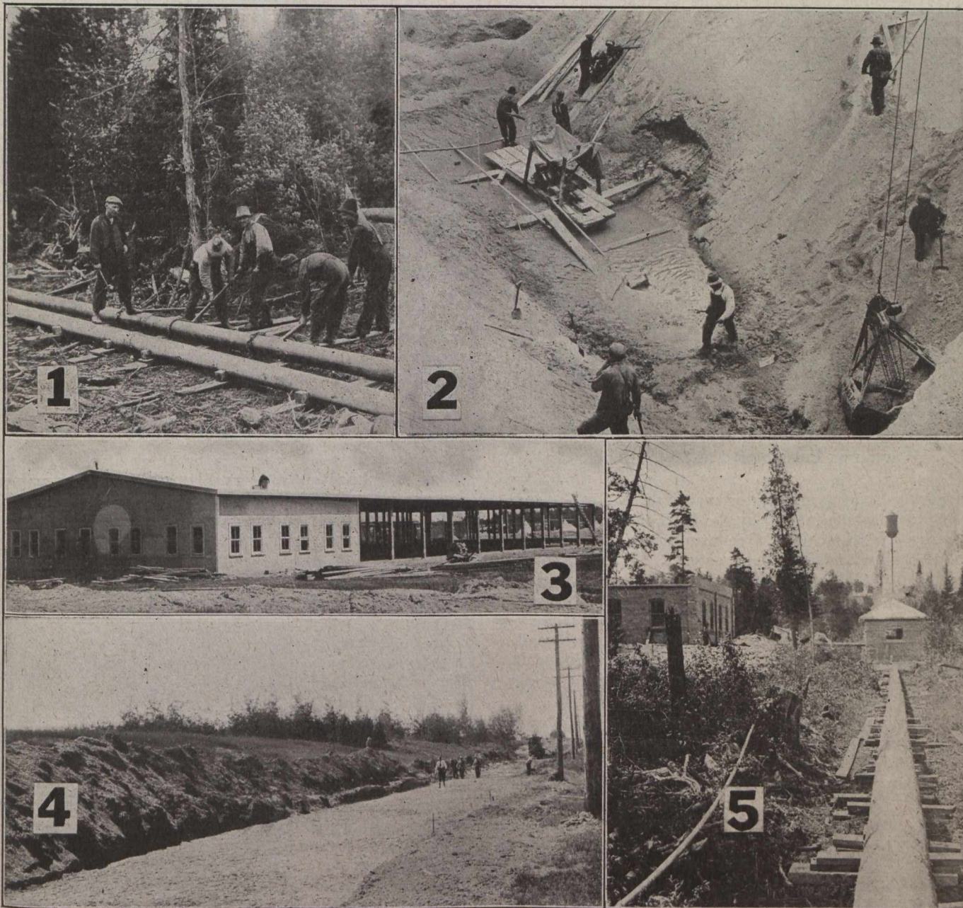
(1) Laying 8-inch Discharge Mains from Pumping Station to Water Tower; (2) Pumping Out Water and Excavating Sand at Site of Sewage Disposal Plant; (3) The Military Garage; (4) Preparing Sub-grade for Concrete Road; (5) View Along Wood Stave Pipe Leading from One of the Wells, with Pump Well and Steel Water Tower in Background, and Pumping Station to the Left of the Pump Well.
