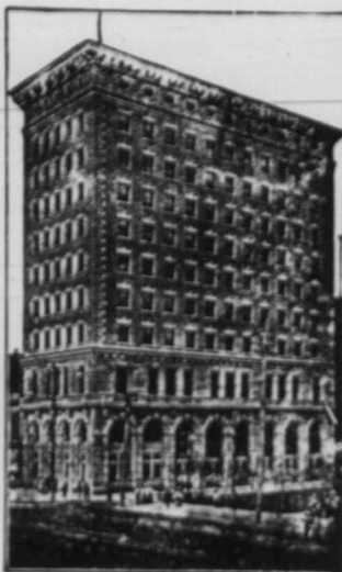
Union Bank Building, Winnipeg
