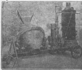
Mixes in Batches. Discharges by Tilting while
