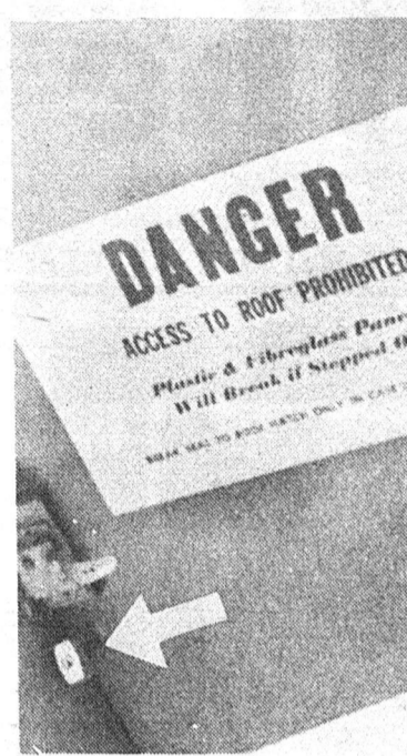
Locked exits Padlocks are clamped on emergency exits to HUB roof.
