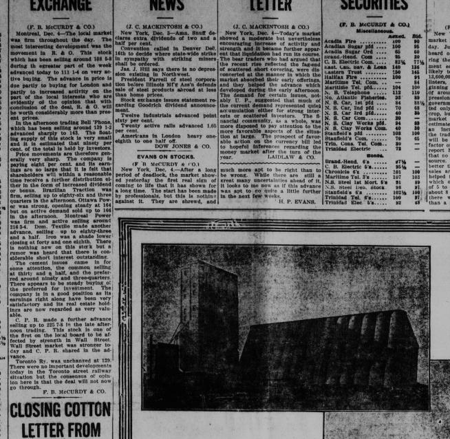
Views of both sides of the million bushel C.P.R. Concrete Grain Elevator at Transcona, Man., which recently settled on its foundations and now stands intact at an angle of 30 degrees.
