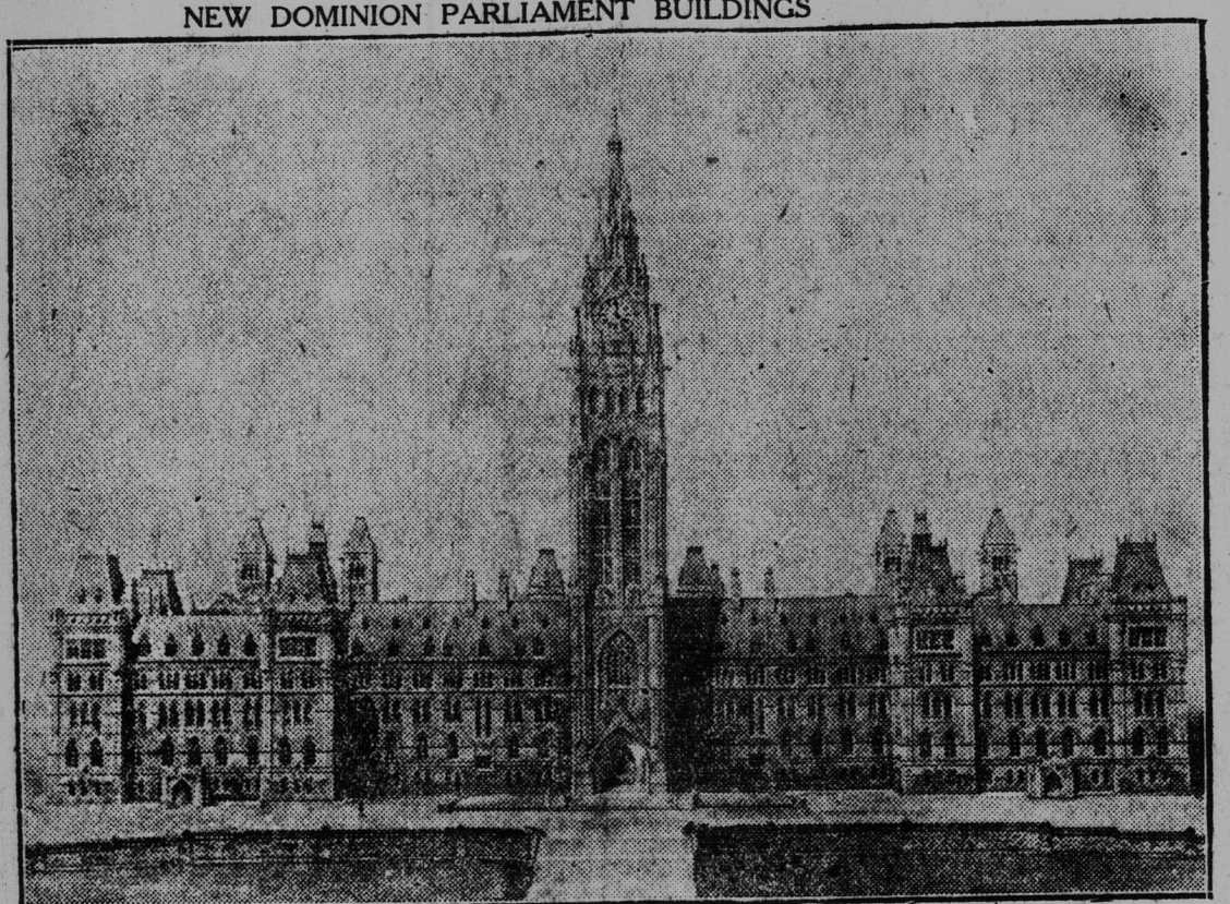
A splendid view of the new House of Commons structure at Ottawa in course of construction.
