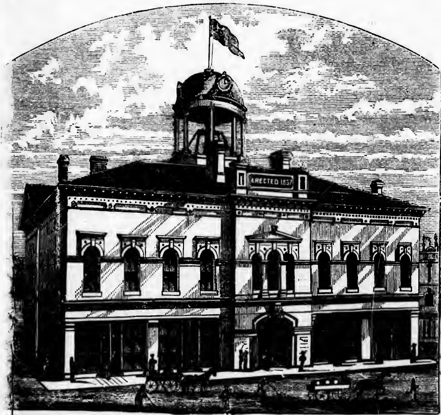
THE TOWN HALL AND MARKET BUILDINGS.
