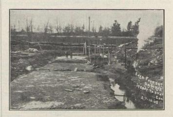
bins, the crusher, and the ends of two tracks connecting with the gravel, pile and cement house. By this means gravel, stone, and cement were handled by the derrick and placed in the receiving bins, or on the platform, as required, and no delay was caused by want of materials for mixing, as the receiving bins held sufficient material for several batches of concrete. The whole of this plant worked very smoothly and systematically, and was very creditable to the designer.
