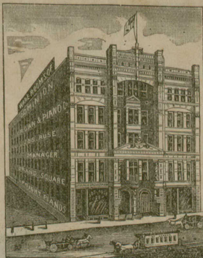
Our Warerooms in course of erection.
