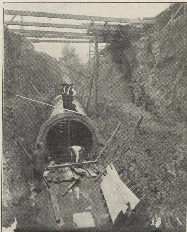
Looking west from Sta. 202, June 16, 1908. Showing mould in place for purpose of receiving concrete.
