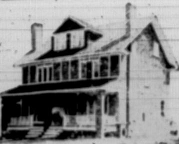
In this Ottawa house Bishopric Stucco Board was used as foundation for all interior plaster and for stucco on exterior walls.
