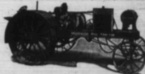
Weight only 600 lbs. Breaks Tread 24 h.p. Draw Bar 12 h.p. Ignition, High Tension Spark Magneto, with Ignition Starter
