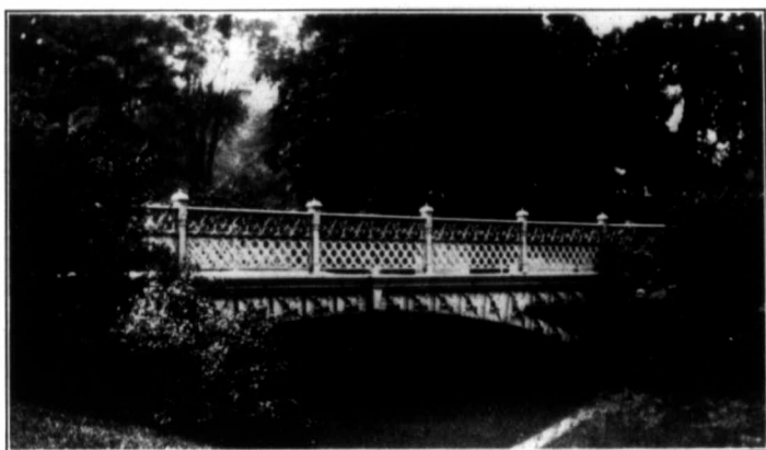
Fig. 7—Bridge in Belle Isle Park, Detroit.
