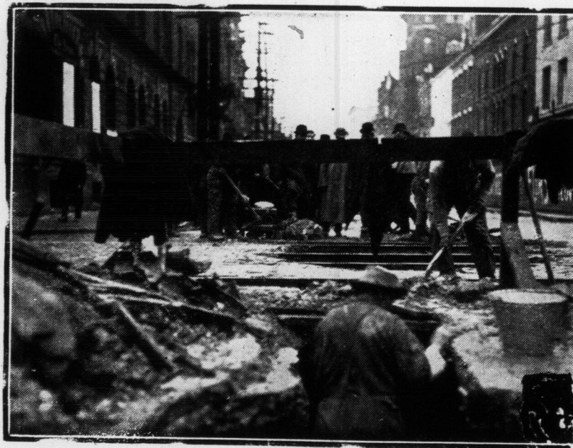
DRILLING UNDERGROUND CHANNELS UNDER DIFFICULTIES. On account of the heavy rains the work of excavating under Yonge and Adelaide-street has been badly hampered, the workmen of necessity having to go slowly for fear of cave-ins.
