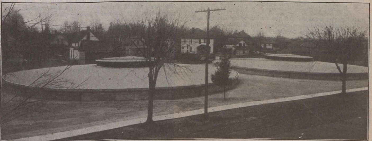
VIEW OF COMPLETED RESERVOIRS AT LEAMINGTON, ONT.
