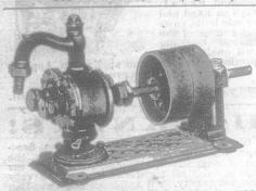
ROTARY FEED PUMP, MOUNTED ON IRON FRAME.
