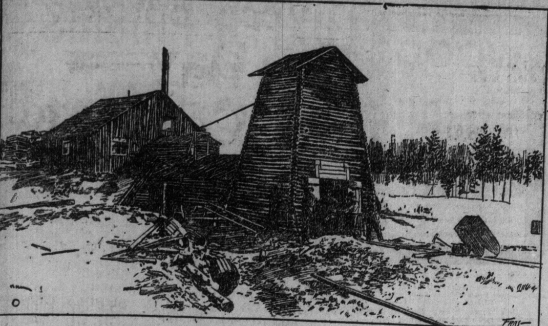
NO. 1 SHAFT HOUSE AT SAW BILL.
