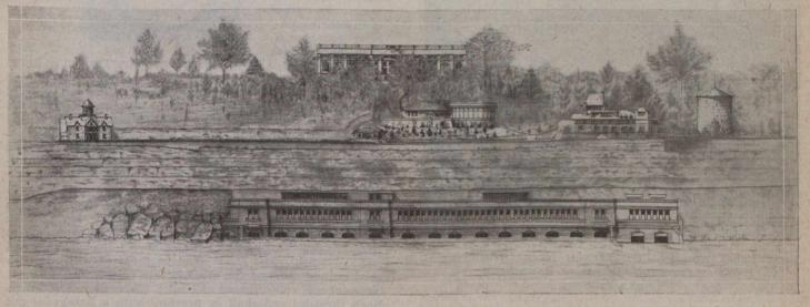
ELEVATION SHOWING POWER HOUSE AT FOOT OF CLIFF—EXTENSION AT THE RIGHT—ON BANK, FROM LEFT TO RIGHT, TABLE ROCK HOUSE, No. 1 AND No. 2 SURGE TANKS, REFECTORY, AND NEW SURGE TANK AT EXTREME RIGHT—ABOVE, DISTRIBUTING STATION
