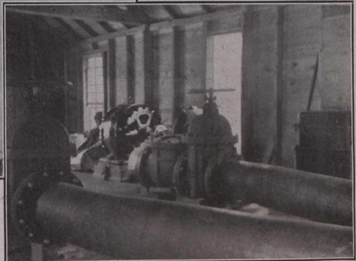
Fig. 1.—Views of COBALT LAKE PUMPING STATION. Two Centrifugal Pumps are Mounted on Scow, Discharging Through Two Flexible Joints.
