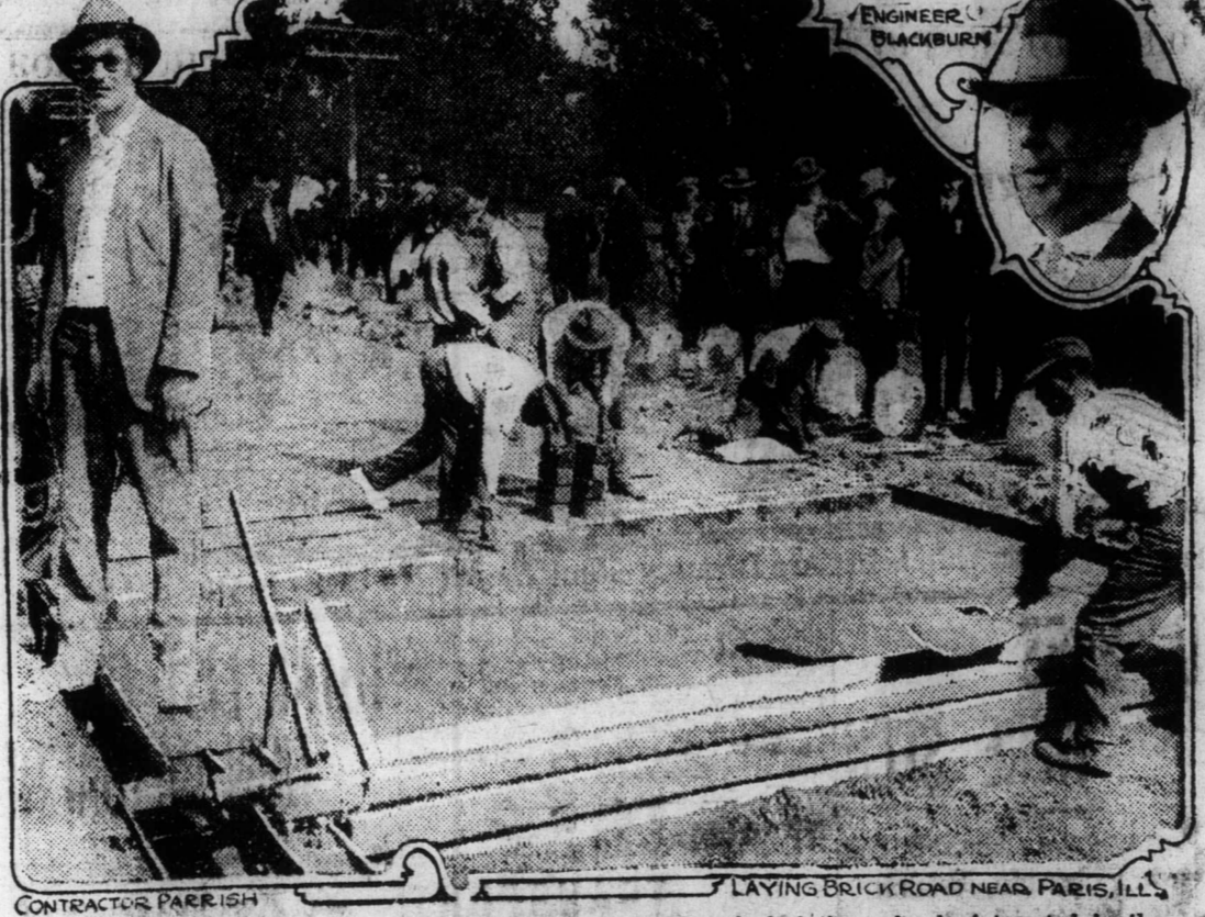
For the first time in the history of road building in America, theory of construction was transferred from the inside meeting place of engineers to the field of practice upon the highway by 300 engineers and contractors when they came together recently at Paris, Ill., to witness the manner and method by which a monolithic brick road is built. The method of laying brick in the green concrete was demonstrated in detail by the execution of every step from the preparation of the roadbed to the completion of the pavement. The machinery used and method of performing the work upon the construction was credited to Engineer W. T. Blackburn and Contractor Alan Parrish, under whose supervision the exhibit was displayed. Among the spectators were members of highway departments of seven states, while representatives from universities numbered more than two score. Editors of engineering journals especially displayed great eagerness in observing details of construction about which they have written in the past so approvingly. Others present were those deeply interested in the economic problem of road building that is now so acute with every user of the highways. All of these visitors expressed a deep appreciation for this unusual opportunity and particularly for the economical methods strongly apparent. The convictions which will be carried back to various sections concerning economy in road building as expressed by many of those present will save to the country 7 thousands of dollars, as a thing seen is believed to be without doubt or foreboding.
