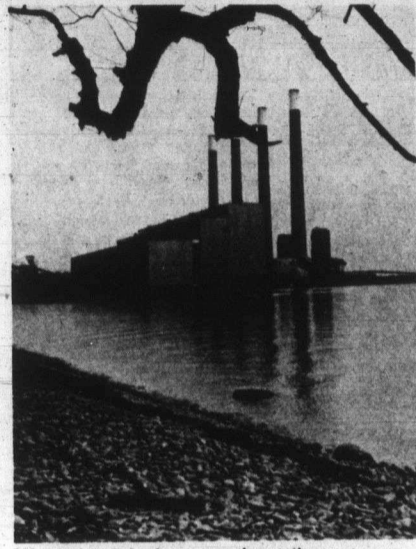
Lakeview generating station.
